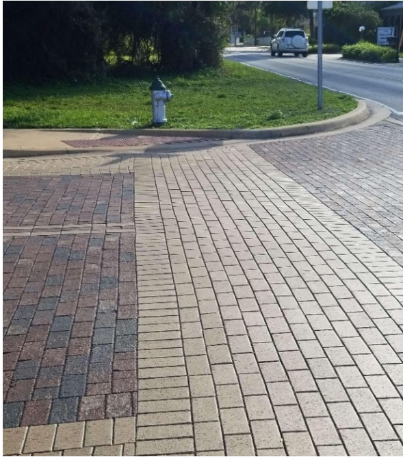
Figure 23: Existing Brick Paver Crosswalk at Milwee Street
