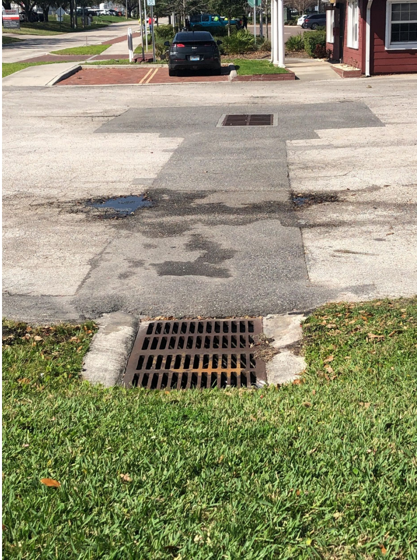
Figure 16: Fire Station Inlets Facing West
