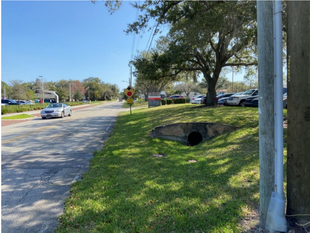
Figure 17: Headwall to South Seminole Hospital Pond Facing East
