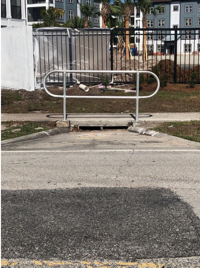
Figure 15: Alta Longwood Connection Facing North
